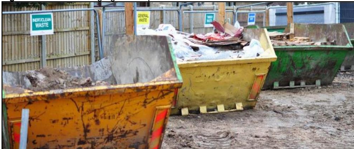
Figure 1 Waste segregation skips
